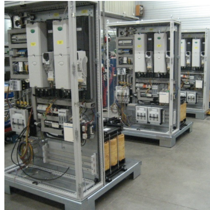
Control cabinets being assembled
